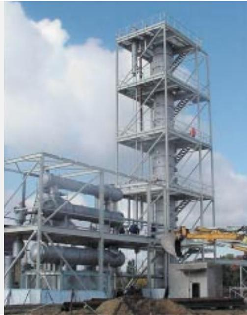
The arrangement shown above, is of a forced circulation reboiler, mounted below the heads condenser and preheater. This plant produces ethanol following the fermentation of the
